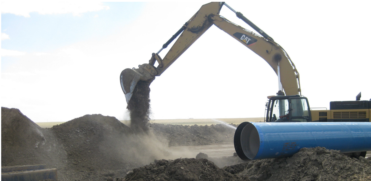
Construction on the Rocky Boy's/North Central Montana Regional Water System.
